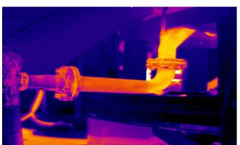
Fig 6: Object temperature, insulation quality condition and energy waste shown using thermography
